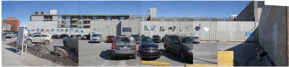
View of parking lot (50/50 corner) - elevation
