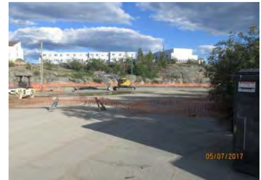
A18 At time of audit, main entrance driveway was under construction.
