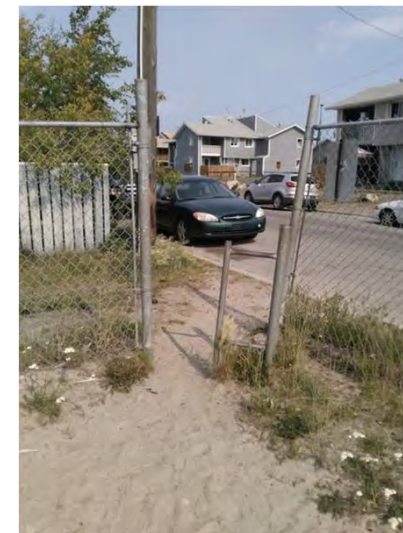
entrance gate impedes access
