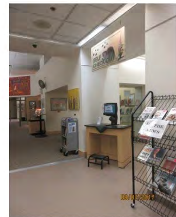
D48 Self-checkout (adj. to circulation desk at front): Potential knee space below, obstructed by furniture). Computer screen height is too high and is for standing users only.
