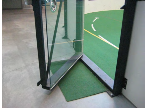
D14 detail access gate/door to soccer fields
