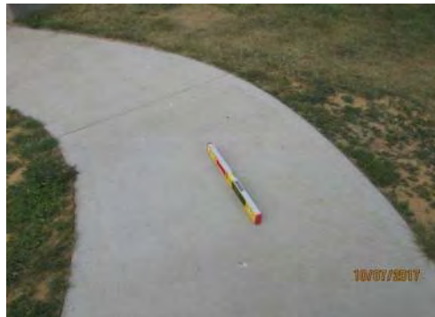
D64 Somba K'e Service Building (exterior): Walkway is narrow. Running slope of walkway to entrance is too steep for users of mobility aids, exceeding 11%.
