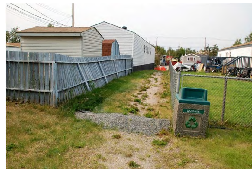
temporary barrier created across access route due to construction
