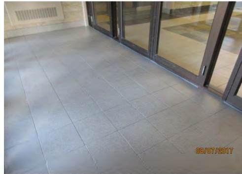
B8 Entrance (stair & ramp, 49th St.): View of vestibule floor space which is limited, when doors swing into space.
