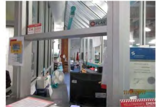
B15 Service counter: Window for communication is cluttered with equipment / supplies. No assistive listening device is provided at service counter for users with hearing loss.
