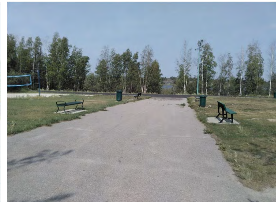
no nearby benches with armrests and backrests access route does not connect to bench base
