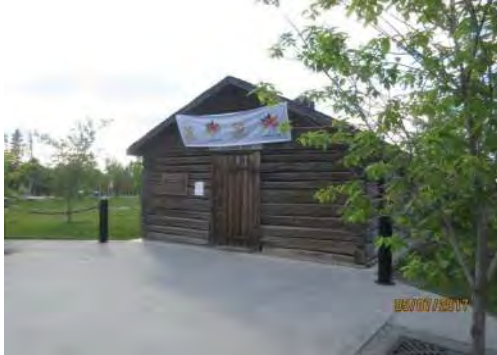
D97 Fireweed Studio (exterior): General view. Building identification signage above entrance is a "rustic" design and is not legible from a distance.
