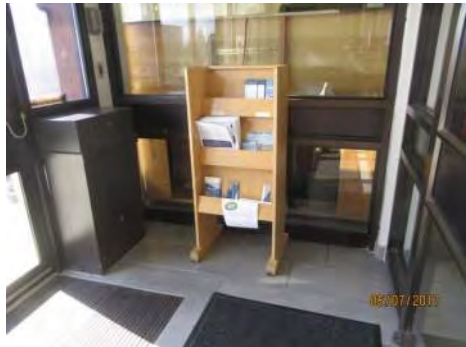
B19 Main entrance (west side): The same information is not provided at accessible entrance or at an adjacent accessible location.
