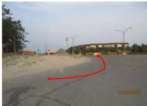
A5 Approach to facility: No separate public sidewalk is provided. Some areas have significant slope.
