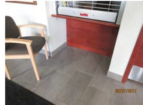
B27 Main Floor, Customer Service Desk: Public Side. No signage identifying availability of assistive listening device for users with hearing loss identified.
