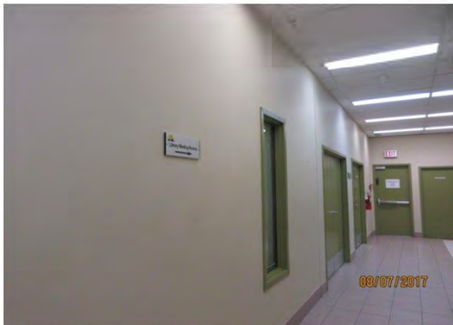
C10 Meeting Room: Directional signage text is too small.
