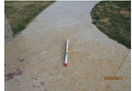
D74 Somba K'e Service Building (exterior): Running slope of walkway to entrance (lower section) is suitable in some areas, for users of mobility aids, at 5% or less.
