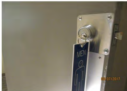
B58 Men's Accessible Washroom: Entrance door is difficult to open, requiring key access. Door is difficult to open.
