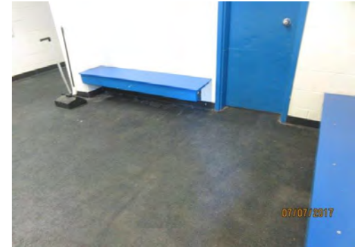
D21 Entrance Lobby / Seating Area (Lower Level): Typical bench seating.
