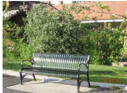
A23 Typical exterior bench seating is accessible. Adjacent clear space on at least one side of benches is not consistently provided.
