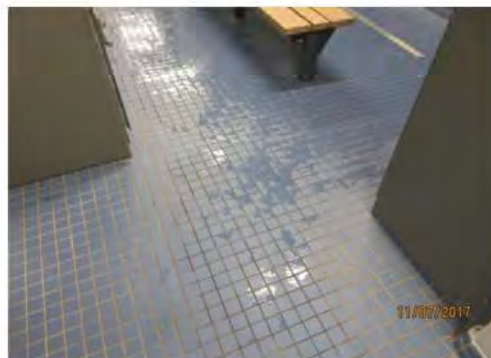
D11 Men's Change Room: Clear width is reduced at entrance, adjacent to lockers.
