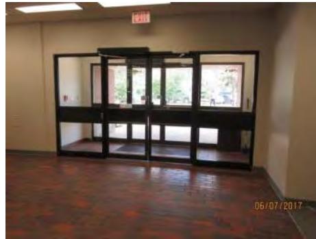
B8 View of interior lobby, accessible entrance (south side). Area is well maintained.
