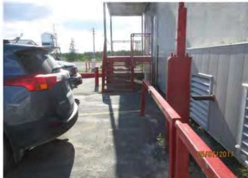
A30 View from accessible parking area looking towards exit stair.
