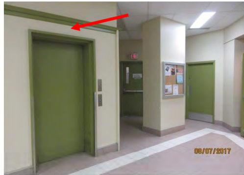
B19 Elevator lobby, 2nd floor. No overhead visual indicator is provided. Floor surface is well maintained.
