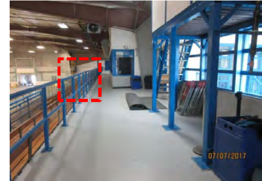
D9 Corridor & Viewing Area (Upper Level, south side): Potential area to accommodate accessible viewing/seating positions.
