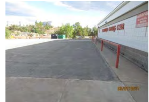
A6 Parking Lot: No spaces are marked. No accessible parking spaces are designated through pavement markings or signage.
