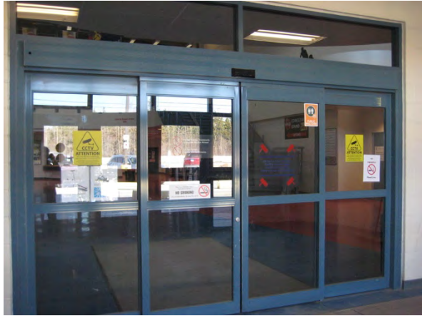
B2 Vestibule – double sliding doors
