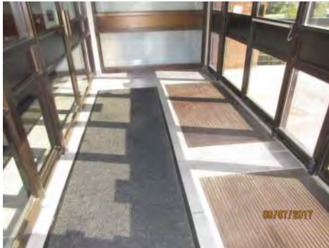
B17 Main entrance (west side): Entrance is not accessible due to stair access only.
