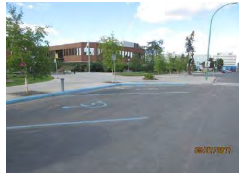
A5 Two (2) accessible on-street parking spaces (angled) are provided on south west side of site. No access aisle and curb ramp is provided and users must travel behind parked cars on roadway.
