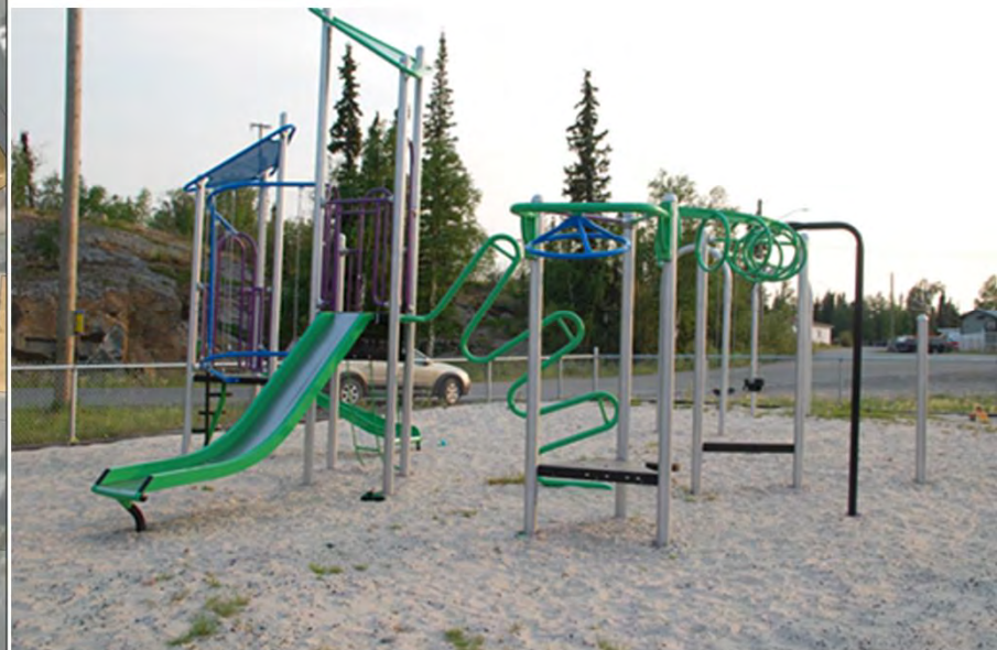
all above ground play equipment is not accessible
