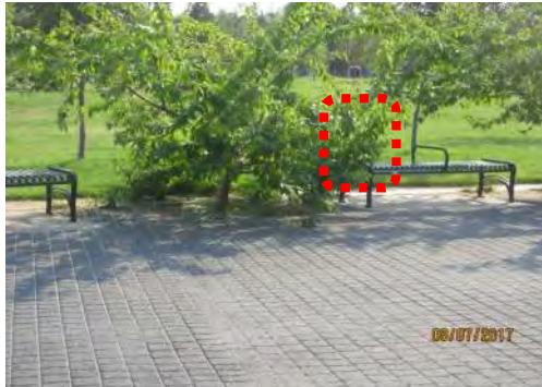
A25 Some bench seating is not accessible, with no back support and adjacent clear space provided on at least one side (e.g., for transfers). Some vegetation also requires maintenance where it obstructs use of bench.
