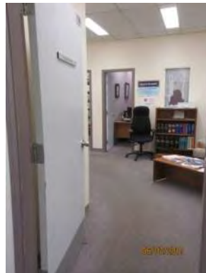
B65 Main floor, Entrance to Human Resources (Room #129): Suitable clear width is provided, however knob door hardware is not accessible.
