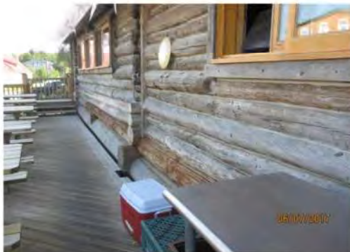
A16 View of exterior deck.
