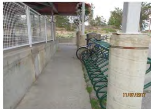
A11 No directional sign is provided to guide users to main accessible entrance. Placement of bicycle rack adjacent to accessible route results in potential bumping and tripping hazard.
