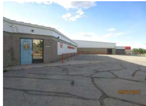
A5 View towards secondary entrance from parking lot. Asphalt appears to be in poor condition in some areas.
