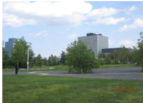
D82 Somba K'e Service Building (exterior): View of adjacent areas.
