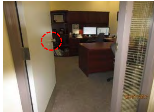
D32 Staff Office, main floor (rear of building): Door clear width is suitable for existing condition. Knob door hardware is not accessible.
