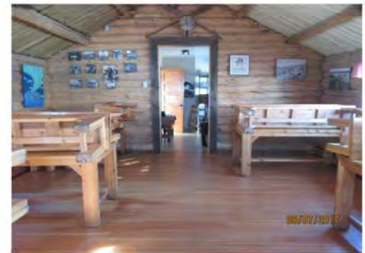
B6 Dining Area: Circulation is suitable for users of mobility aids. No accessible seating position was identified for tables.
