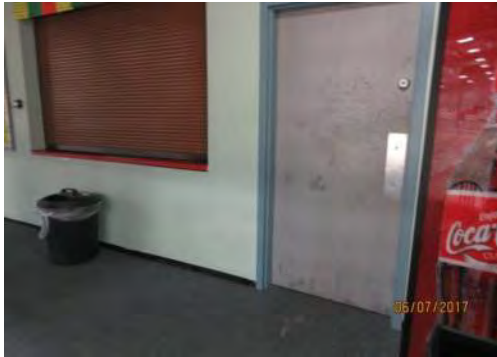
D31 Concession / Serving Window (lower level): Serving counter is mounted at standing height. Space appeared to be under renovation.
