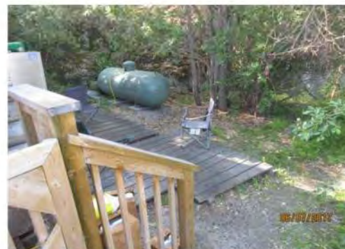
A23 View of exterior staff area: Stepped access only, off of exterior deck.
