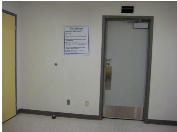
B9c Door to adjoining washroom from main level change room.
