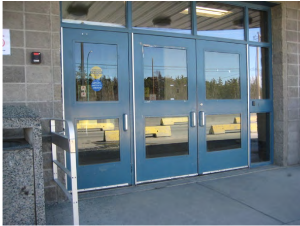
B1 Main entrance doors
