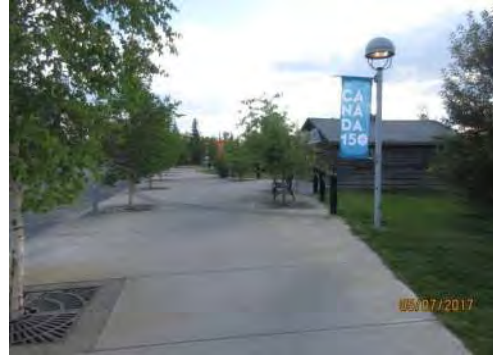
D98 Fireweed Studio (exterior): Ample clear width is provided along pedestrian sidewalk, leading to and from studio.
