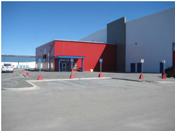
A3 accessible parking stalls near main entrance
