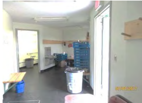
D86 Somba K'e Service Building (interior): Many interior areas are used for storage. Clear floor space is limited.
