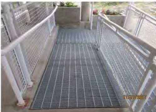
A22 View of ramp, from top landing and main entrance area. Extensions at top landing are not provided but would also be potential bumping hazards.
