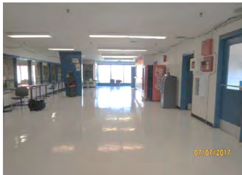
B11 Enclosed Viewing Area and Entrance Lobby (looking north): Generally, area is well maintained for circulation. Some glare is reflected from flooring surfaces, adjacent to window wall.
