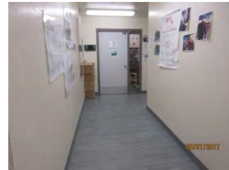
B60 Main floor, corridor (adj. to Office #118): Suitable clear width is provided.
