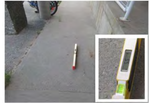
A15 Approach to main entrance from accessible parking spaces (top section): Running slope is on-compliant at 5.5%.
