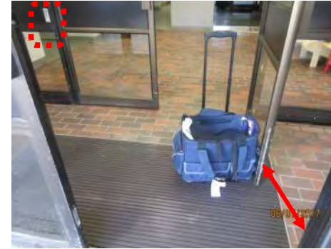
B3 Accessible entrance (south side): Floor space is limited for interior vestibule, including space between two doors in series.
