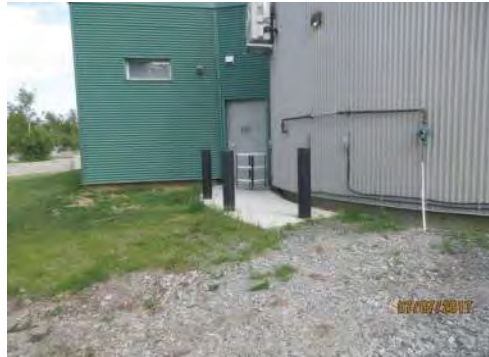
D61 Somba K'e Service Building (exterior): Approach to storage and utilities areas.
