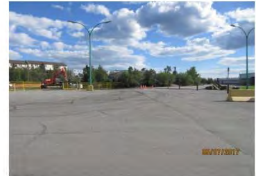
A3 View if main parking lot. Drive aisles are not clearly marked. No clearly marked or designated pedestrian walkways.
