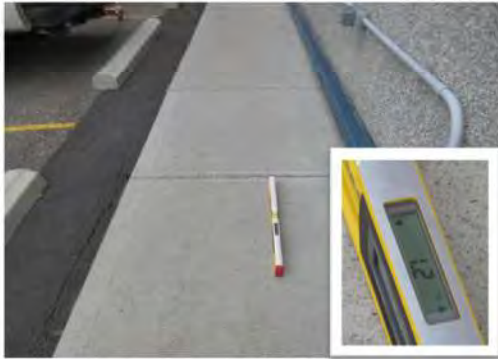
A24 Approach to staff entrance / exit (east side): Running slope is suitable at 1.2%.
