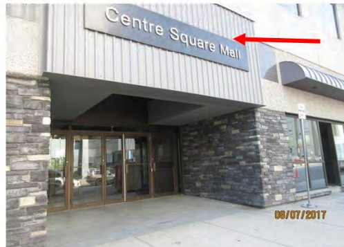
A22 Mall Entrance: Sloped route is provided, however, running slope is non-compliant. Power door operator is provided. Accessible entrance door is not marked with International Symbol of Accessibility decal.
