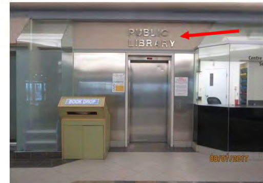
C24 Book Return, elevator lobby (ground floor, mall): Identification sign has large print and suitable colour contrast. Overhead library identification signage does not have strong colour contrast.
