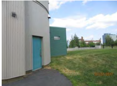
D83 Somba K'e Service Building (exterior): Approach to storage and utilities areas.
