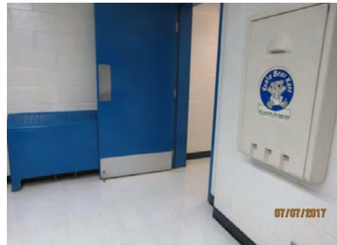
B23 Women's Accessible Washroom (Upper Level): Entrance doors have limited clear width but typically suitable for an existing condition.
