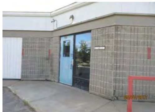
A10 Secondary entrance: Marked as "Concession" entrance. Level access is provided for users of mobility aids. Entrance is not marked as accessible through signage.
