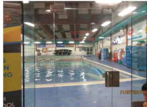
B11 Viewing Area: Glazing is not marked to prevent potential bumping hazards especially for users with vision loss. Glass entry/exit door and adjacent glazing is difficult to identify, especially for users with vision loss.
