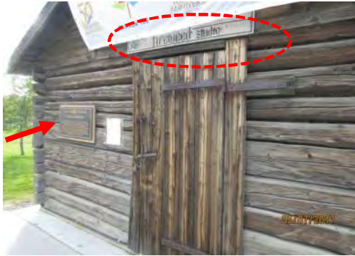
D103 Fireweed Studio (exterior): Building identification signage is "rustic" design, with no accessibility features. Interpretive plaque signage has limited to no accessibility features, mounted adjacent to entrance.
