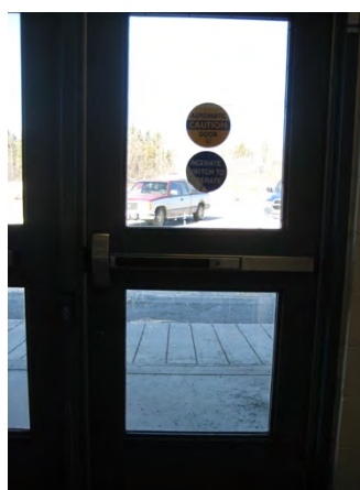
C6 decals on main entrance door
