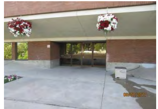
A18 Accessible walkway, to accessible entrance (south side), is in very good condition and surface is well maintained. No problems were identified.
