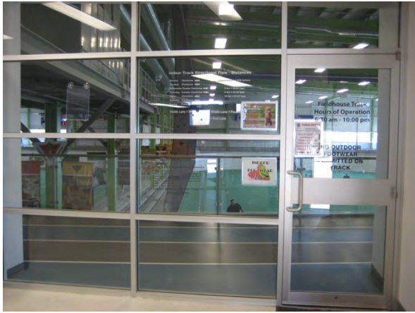
D19 door and glazed partition to walking track in upper level lobby area.
