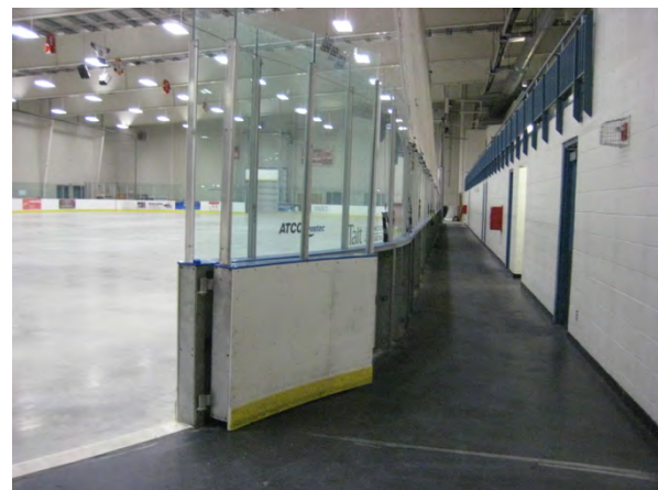
D11 ice access door and one side of perimeter corridor (typical)
