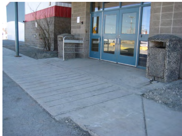
A6 Main entrance doors
