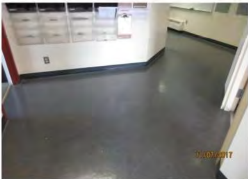
B23 1st floor, entrance vestibule: Circulation is suitable.
