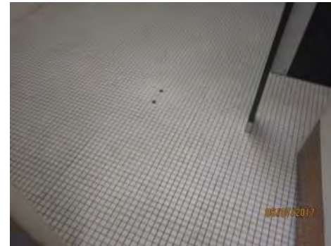
B108 2nd Floor, Men's Accessible Washroom (Staff): Clear door width is non-compliant. Awkward configuration at entrance due to privacy partitioning.
