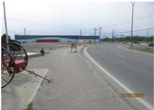
A3 Franklin Avenue: Pubic sidewalk (north east side of site).
