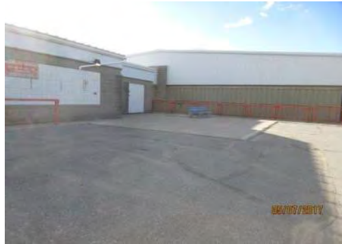
A1 View towards main entrance from parking lot. No accessible routes are typically provided due to high transitions between parking surface and concrete walkways.
