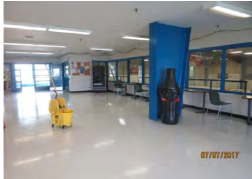
B13 Enclosed Viewing Area and Entrance Lobby (looking south): Ample clear floor space for circulation is provided. Strong colour contrast is provided on surfaces of support column.
