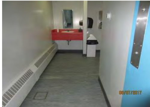
B37 Main Floor (adj. to entrance): Women's Washroom. Identified as accessible through door signage but it is not accessible.
