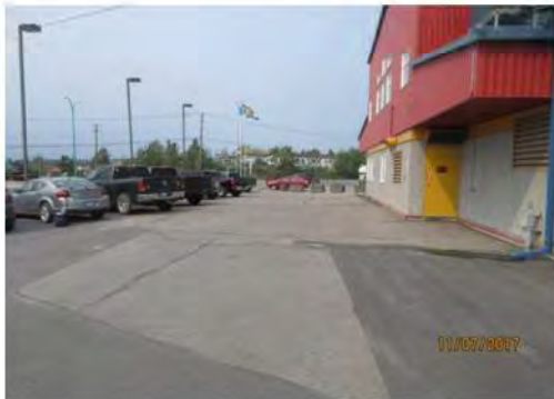
A10 View from Taylor Road: Approach to main entrance. No separated or marked accessible pedestrian route is provided.
