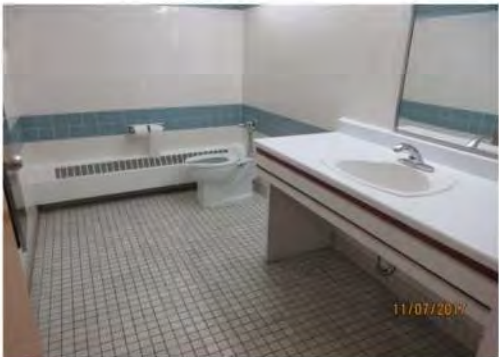
B34 2nd floor, interior view of Washroom #1: No accessibility features identified. However, 2nd floor is not accessible.
