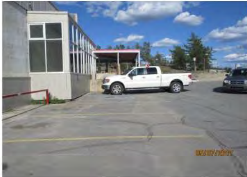
A7 Only some parking spaces are marked.
