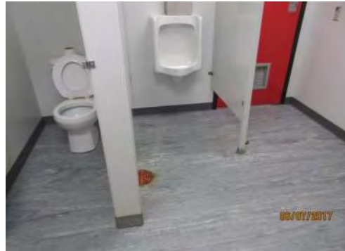
B50 Main Floor (adj. to secondary entrance): Men's Washroom. Identified as accessible through door signage but it is not accessible.
