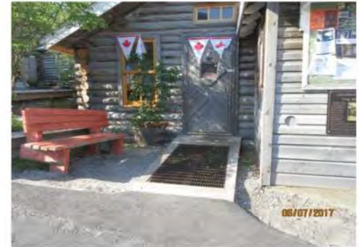
B3 Approach to main entrance, off of Racine Road, with gently sloped transition.
