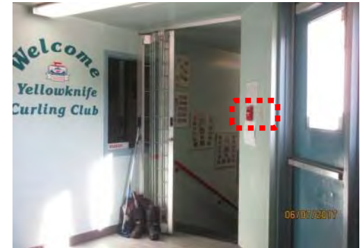
C6 Typical fire pull and light switch are mounted too high for users of mobility aids.
