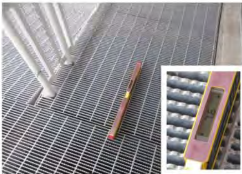
A24 Ramp, intermediate landing : Running slope is suitable at 7.6%.
