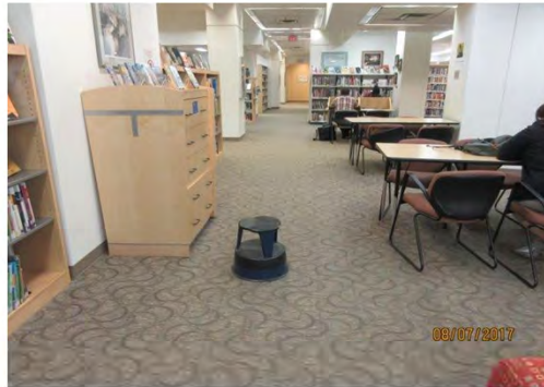
B37 Central circulation route (between Adult & Kid Sections): Temporary obstruction for users of mobility aids due to portable step located in aisle.
