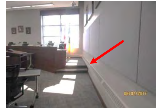
D15 Council Chamber: Approach to upper seating level from Staff Seating Area. Step access only.
