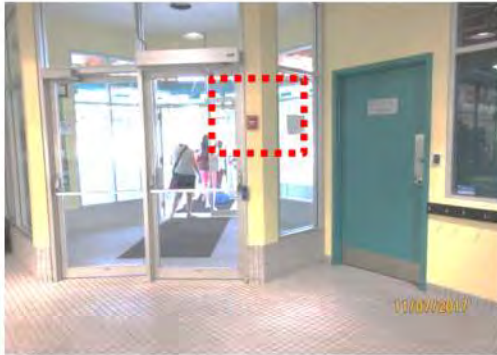
B7 View of approach to main entrance and entrance to Office.
