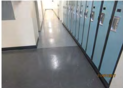
B24 1st floor, view of central corridor and staff locker area: No accessible lockers provided / identified.
