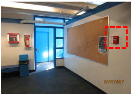
C4 Fire alarm pull, Lower Level: Mounted too high for users of mobility aids. However, there is no elevator access to lower level at this time.
