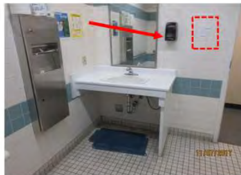
B41 1st floor, Unisex accessible washroom: Occupancy sensor provided. Lavatory & mirror are accessible. No pipe protection below. Soap dispenser is mounted too high. Paper towel dispenser is too high & operating control is not accessible.
