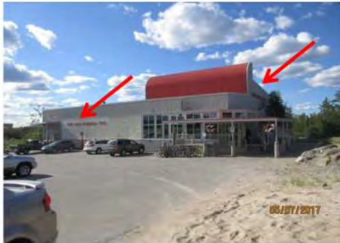
A1 Approach to facility: No separate public sidewalk is provided from site boundary to main entrance. Some areas of parking lot have significant slope. Building identification signage has strong colour contrast. Exterior site and facility identification signage is limited.
