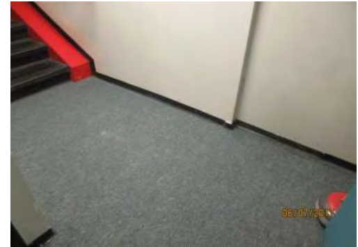
B27 Stair #1: View of landing area (lower level).
