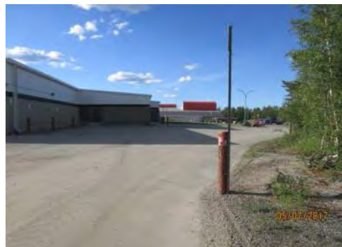
A17 No sidewalk is provided off of main entrance driveway and from site perimeter, off of 50 Avenue.
