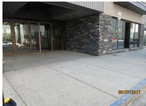
A23 Mall Entrance: Sloped route is provided, however, running slope is non-compliant.
