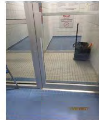
D3 Entrance to Change Room vestibule, from Staff work area (adj. to Pool): Floor space is very limited on both sides. Pull-plate door hardware is not accessible. Door clear width is limited.
