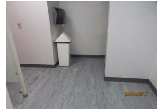
B51 Main Floor (adj. to secondary entrance): Men's Washroom. Identified as accessible through door signage but it is not accessible.
