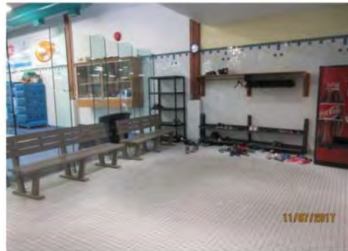
B8 Viewing Area: No arm rest options provided for bench seating. Seating surface is typically too low.
