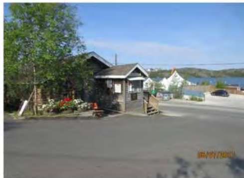
A5 No separated pedestrian route / public sidewalk is provided.
