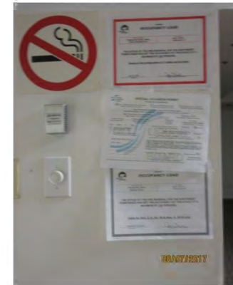
C15 Light switch is mounted too high and requires twisting of wrist to activate. Posted signage is cluttered.
