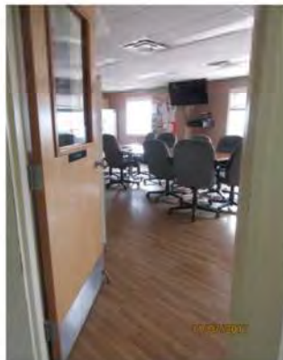
D10 1st floor, Kitchen, view from entrance #1: No accessibility features identified. However, interior floor space is open concept and potential accommodations can be made.
