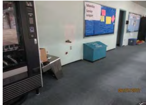
D32 Lower Level: Drinking fountain was not in working order and was not wall-mounted. Vending machine controls are not accessible.
