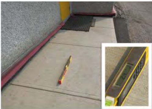
A14 Main entrance area: Running slope is suitable at 2.4%.
