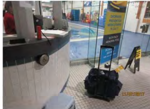
B14 Service counter: No accessible counter provided. At time of audit, power door operator was not turned on when tested by activating PDO control.
