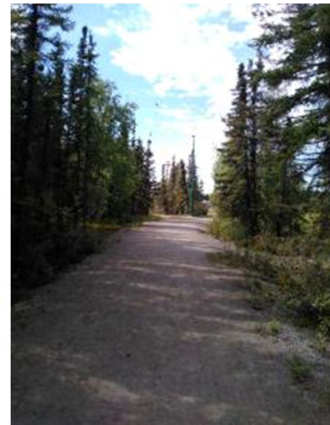
Typical trail compact gravel surface
