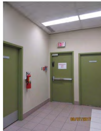
B77 Exit Stair (adj. to Meeting Room): Assumed alarm is activated when door is opened as signage indicates "emergency exit only". Stair was not reviewed.
