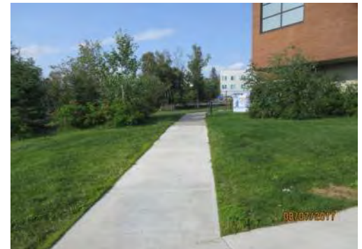
A30 Accessible walkway (view from north west side of site). No problems were identified.
