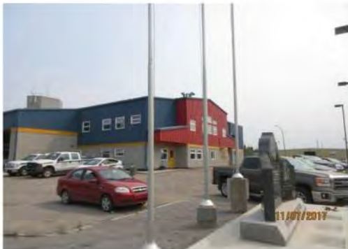
A27 View of facility from public sidewalk and approach (north east side).
