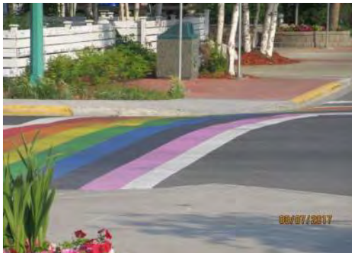
A16 No tactile walking surface indicators typically provided at curb ramps at pedestrian crosswalks.
