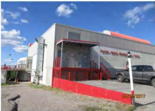
A29 View looking towards exterior deck and patio area at rear of facility. View of exit door.
