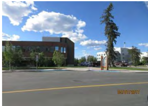
A4 One (1) accessible on-street parking space (angled) is provided on south east side of site. No access aisle is provided. Curb ramp is blocked when vehicle is parked.
