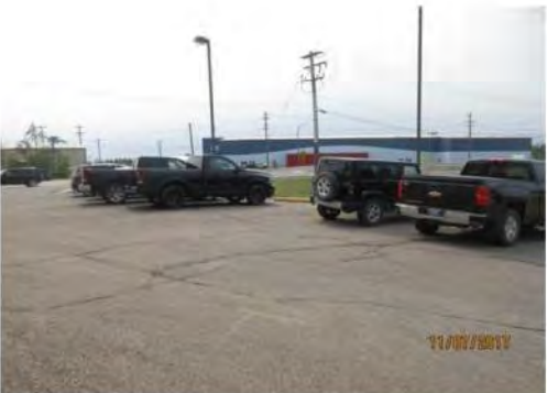
A5 Public and staff parking lot, north side of site. No accessible parking spaces identified.
