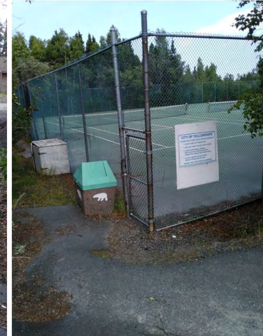
trail from laneway includes a steep drop limited room to manoeuvre at the entrance gate
