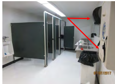
B29 Men's Accessible Washroom (Upper Level): View of interior floor space for circulation. No accessible lavatory is provided with knee space clearance below. Amenities are typically mounted too high (hand dryer & baby change tables).
