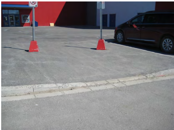
A5 curb ramp and signs marking access route
