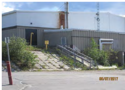
A16 View of stair system, from exit door (north side). Wooden stair generally does not meet current requirements including oversized wooden handrails. Level access is not provided at exit door (multiple level changes when exiting).
