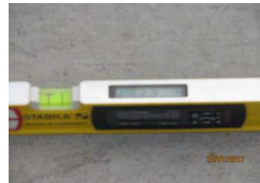
D71 Somba K'e Service Building (exterior): Cross-slope is too steep at some sections, exceeding 2%.
