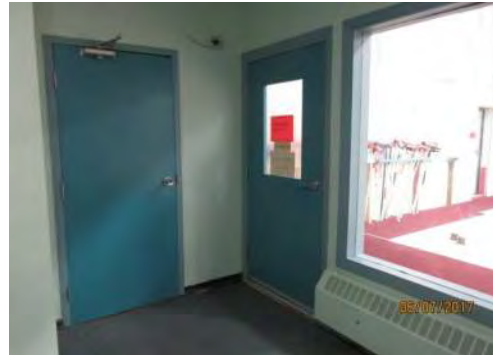
D20 Entrance to curling rink from viewing area.
