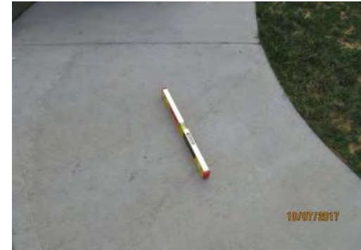
D68 Somba K'e Service Building (exterior): Running slope of walkway to entrance (upper section) is too steep in multiple sections, for users of mobility aids, exceeding 9%.
