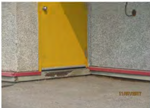
A11 Emergency Generator Room: Stepped exit / entry.
