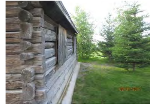
D105 Fireweed Studio (exterior): General view.
