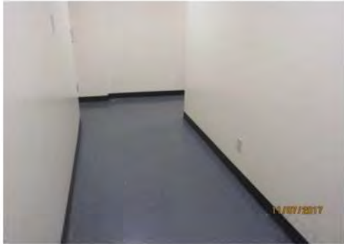
B31 1st floor, typical corridor, adjacent to Dormitory: Generally suitable clear width is provided for circulation, and low level of use based on size and occupancy of this facility.
