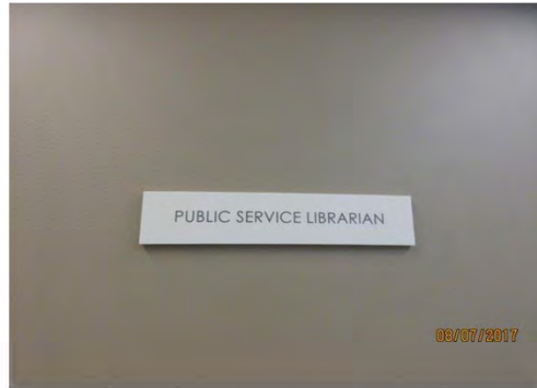
C8 Office identification Signage (Typical): Colour contrast is suitable. Print size is typically small, with no braille / tactile features or alternate accessible signage provided.
