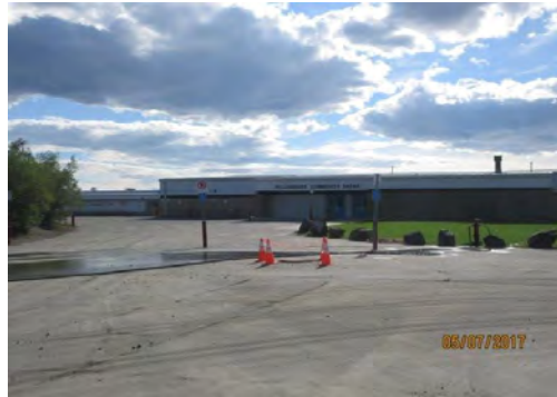
A1 Approach to main entrance, from west side. Parking spaces are not clearly marked (e.g., pavement line markings), including accessible parking. No separated or marked accessible pedestrian route is provided from site boundary, leading to main entrance.
