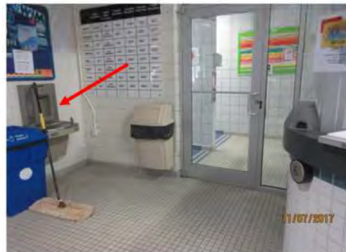
C5 An accessible drinking fountain is provided adjacent to service counter but may be difficult to identify due to limited signage. Approach is temporarily obstructed by placement of recycling bin and cleaning equipment.
