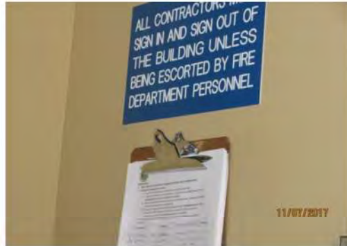
C1 Main entrance lobby, informational signage and sign-in clip-board: No accessibility features identified.
