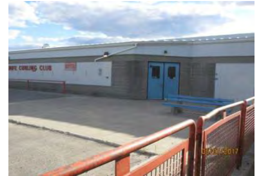
A3 No curb ramp is provided. Transition between parking area and sidewalk leading to main entrance is too high for users of mobility aids.
