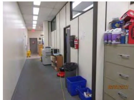
B44 2nd floor corridor (south side): Clear width and circulation is obstructed by temporary storage of items.
