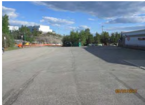
A4 Parking Lot: No spaces are marked. No accessible parking spaces are designated through pavement markings or signage.
