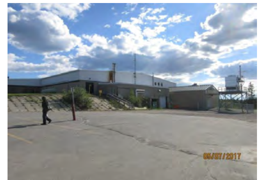
A15 View of stair system, from exit door (north side). General view of exterior conditions adjacent to exit as well as entrances to storage facilities.
