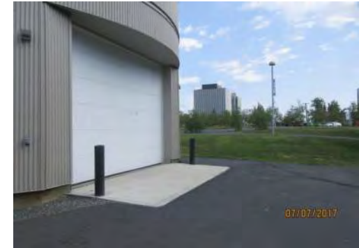
D62 Somba K'e Service Building (exterior): Garage entrance door at rear of building.
