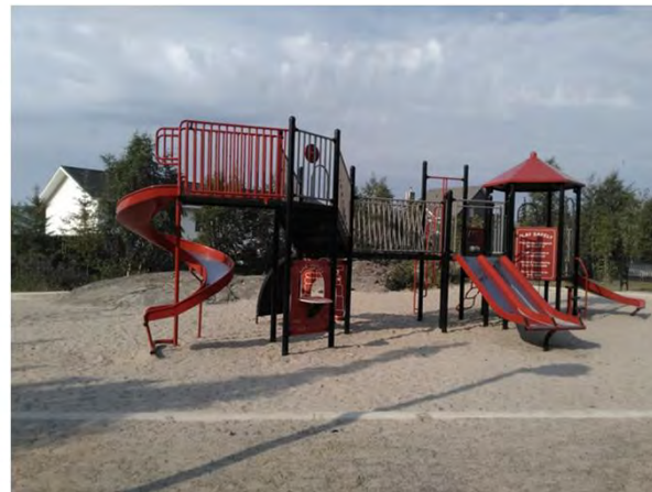
playground equipment is not accessible
