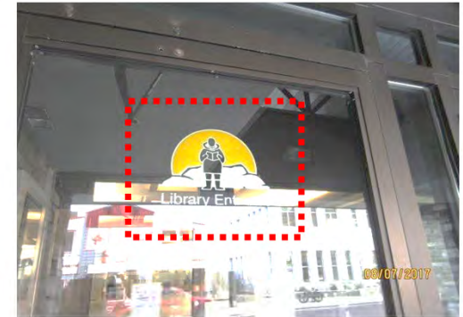
A3 Library entrance is marked with door identification signage (e.g., decal), however, it is difficult to identify from a distance.
