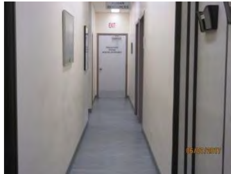
B68 Main floor corridor (east side, adjacent to HR): Clear width is provided, however, it is limited.
