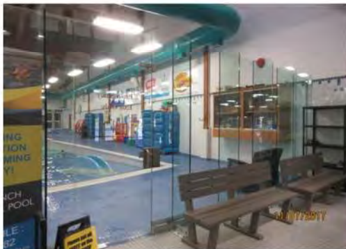
B10 Viewing Area: No arm rest options provided for bench seating. Potential rest area and transfer space beside bench is temporarily obstructed by signage.
