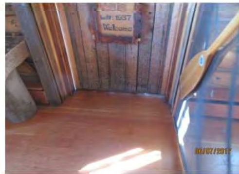
B5 Main entrance: Suitable clear width is provided.
