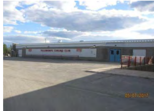
A2 View towards main entrance from parking lot. No accessible routes are typically provided due to high transitions between parking surface and concrete walkways.
