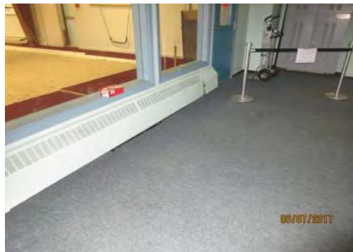
D10 Curling Rink Viewing Area (lower level): View of floor space provided.
