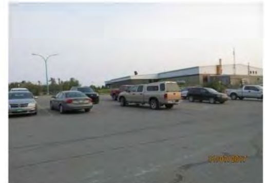
A6 View if main parking lot. Generally, parking space markings have faded.
