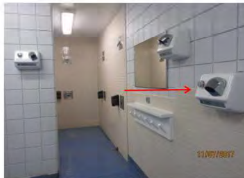
D23 Men's Change Room: Approach to shower stalls (multiple occupancy). Lowered, automatic hand dryer is provided.
