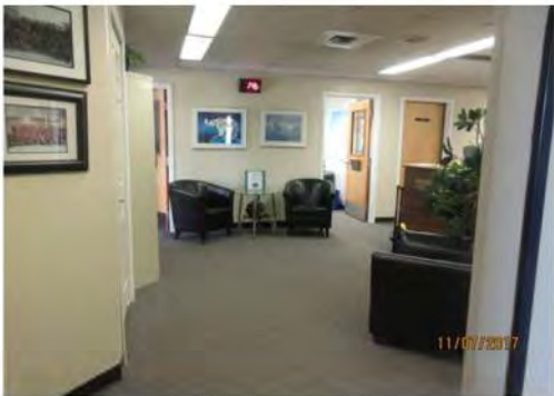
B14 2nd floor, entrance lobby & reception area: Circulation is suitable. No elevator access is provided to 2nd floor.
