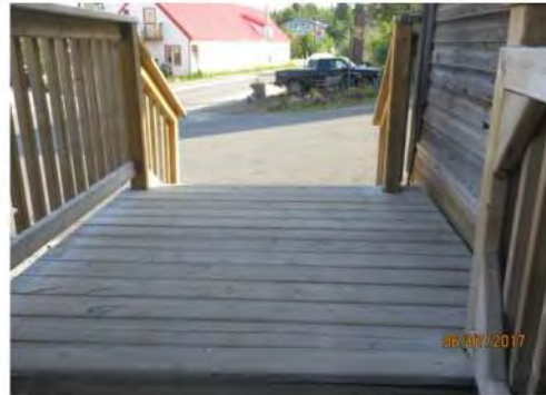
A14 View of exterior deck (top landing of stair).
