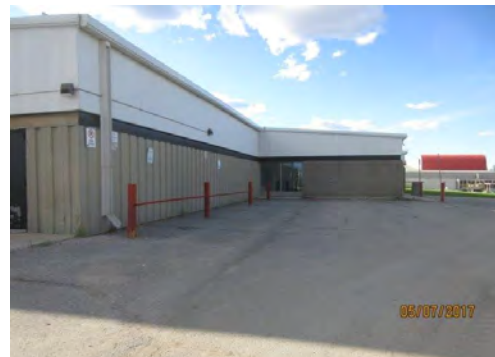
A5 No parking spaces are marked (south side of site). No separated pedestrian routes are provided from site boundary.
