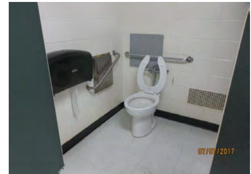
B24 Women's Accessible Washroom (Upper Level): Stall floor space is limited. Flush control is not on transfer side of toilet. Stall doors are not self closing. No L-shaped grab bar is provided at side of toilet. Toilet paper dispenser mounted too far and too high.
