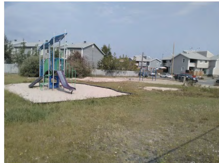
play structures are not accessible retained sand limits accessibility
