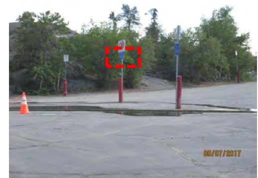
A3 Approach to main entrance, from west side. Accessible parking spaces are marked with post-mounted signage only, which is damaged / obstructed. No separated or marked accessible route is provided (e.g., directional signage), leading to main entrance.
