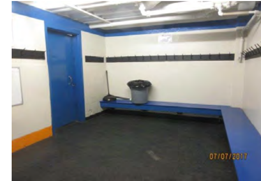
D54 Change Room #1 (Lower Level, south side): Typical change room conditions.
