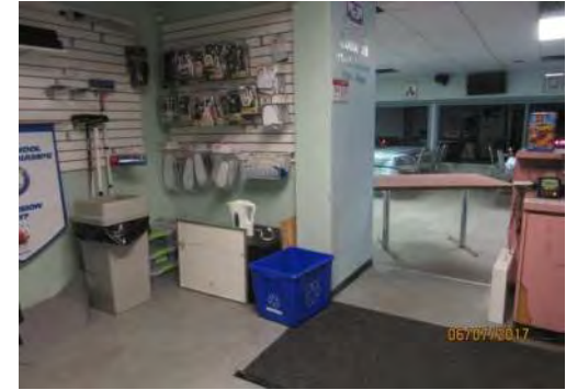
B15 View of Pro-shop area, upper level (adjacent to Concession Stand / Bar). Generally, no accessibility features identified (e.g., mounting heights for retail displays etc.).
