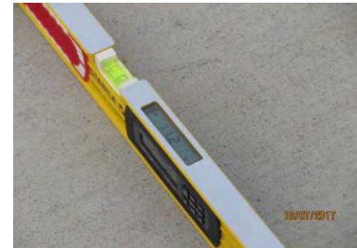
D65 Somba K'e Service Building (exterior): Running slope of walkway to entrance is too steep in multiple sections, for users of mobility aids, exceeding 11%.
