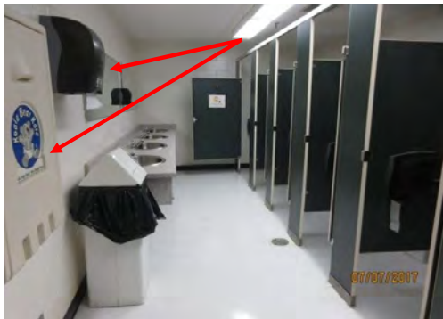
B22 Women's Accessible Washroom (Upper Level): No accessible lavatory is provided with knee space clearance below. Amenities are typically mounted too high (hand dryer & baby change tables).
