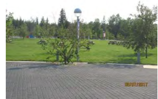
A27 Typical picnic tables in background are not accessible and are not provided on or as part of accessible route (e.g., placed on grass surface only).
