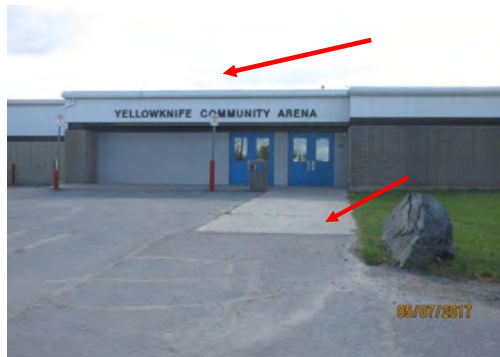
A4 View of facility identification signage. Generally, no directional signage is provided throughout site to guide users to main entrance. Transition from separated accessible pedestrian route and drive aisle (asphalt surface) is not marked with TWSI.
