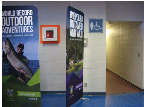
B20 AED Cabinet to left of washroom entry.
