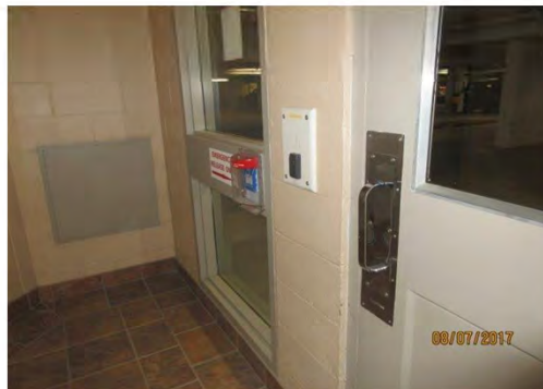
B52 Elevator lobby, parking garage: Door was secured at time of audit.
