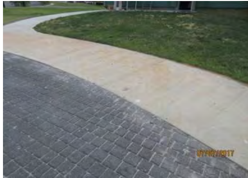
D79 Somba K'e Service Building (exterior): View of approach to walkway that leads to entrance of facility. Walkway is narrow.
