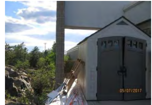
A15 View of south side of building.
