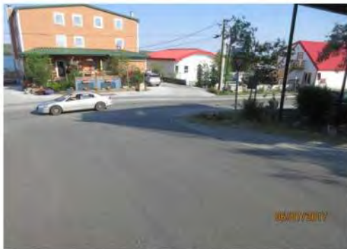
A4 No separated pedestrian route / public sidewalk is provided.
