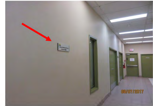
B21 Main corridor, 2nd floor: Corridor clear width is suitable. Directional signage is provided, however, text size is small. Floor surface is well maintained.
