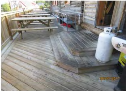
A19 Secondary entrance (side): Stepped access only.
