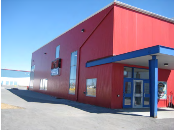
A1 Main façade and entrance canopy
