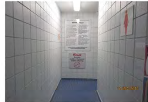
D9 Entrance corridor to Women's Change Room . Clear width is typically limited for larger wheeled mobility aids. Identification signage is not accessible.
