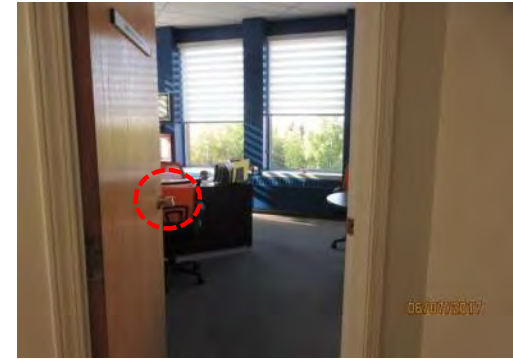
D42 Director of Planning, 2nd floor (Room #222): Entrance is non-compliant with less than 800 mm clear width and knob door hardware.
