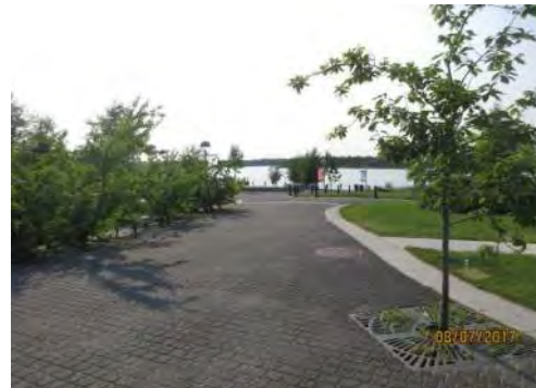
A29 Approach to waterfront (south west side). No problems were identified.
