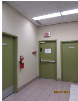
C17 Exit Stair (adj. to Meeting Room): Assumed alarm is activated when door is opened as signage indicates "emergency exit only". Stair was not reviewed.
