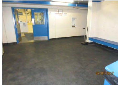
D20 Entrance Lobby / Seating Area (Lower Level): Potential area to accommodate elevator provision.
