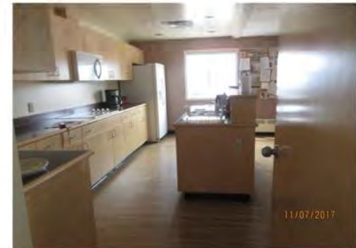
D12 1st floor, Kitchen: No accessibility features identified.
