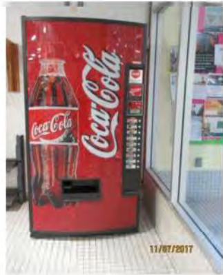
C1 All operating controls are not accessible for existing vending machine (e.g., some upper controls exceed 1200 mm max).
