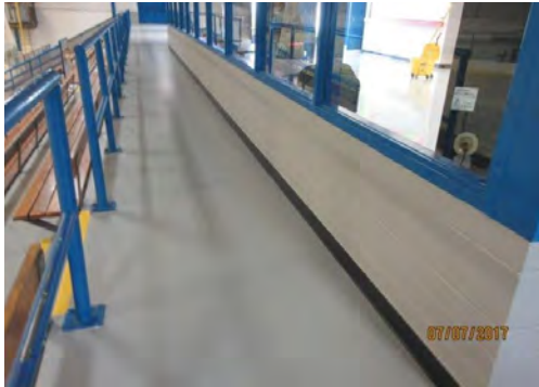
D13 Corridor (Upper Level, north side): Suitable clear width is provided, although it is limited to allow one way traffic only.
