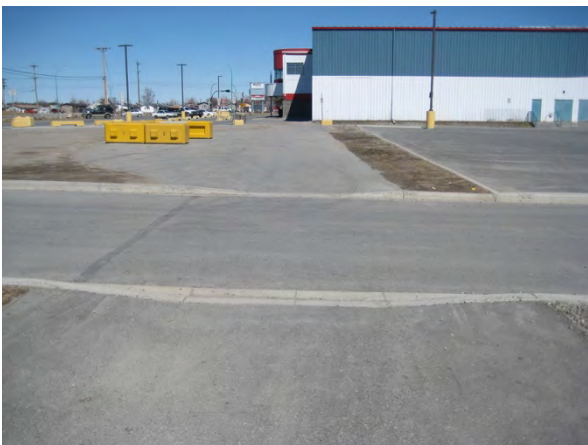
A5 Pedestrian crossing route
