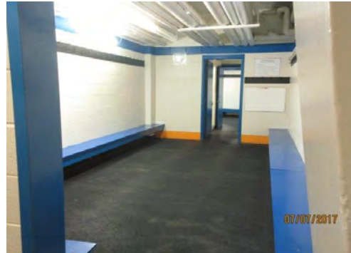
D32 Change Room #3 (Lower Level, north side).
