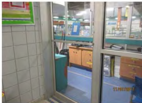
D4 Entrance to staff work area: Floor space is very limited. Door hardware is push bar type (door swings into room).
