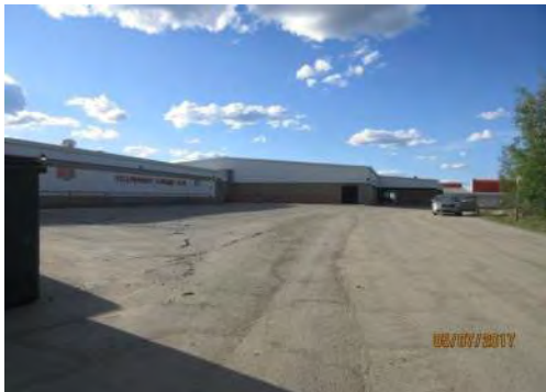
A16 No sidewalk is provided off of main entrance driveway and from site perimeter, off of 50 Avenue.
