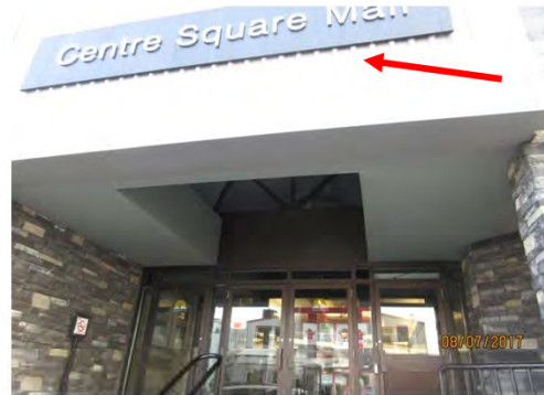
A2 Library entrance, via stair & ramp access, off of 49th Street. Building identification signage on façade is prominent with large text and suitable colour contrast.
