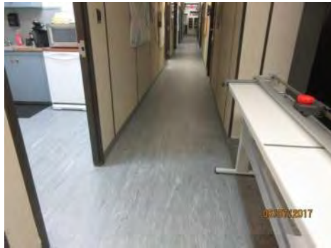
B73 Main floor, corridor adjacent to Staff Kitchen. Equipment projects into clear width of accessible route.
