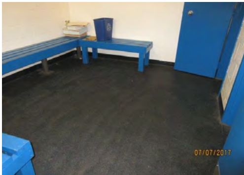
D28 Referee's / Official's Change Room (Lower Level, north side).
