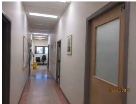
B41 2nd floor corridor (typical). Corridor is well maintained. Clear width is suitable.
