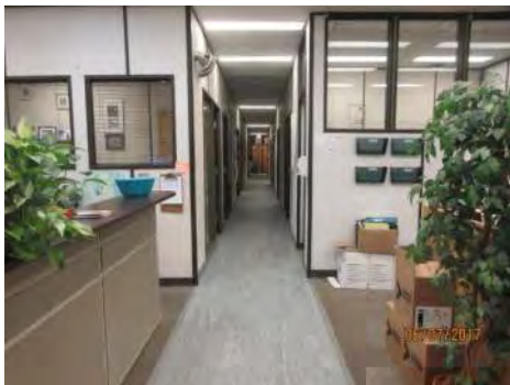
B70 Main floor, Community Services reception area (south east side): No lowered counter is provided.
