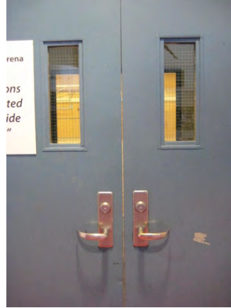
B15 Door hardware and vision panels
