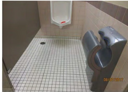
B62 Men's Accessible Washroom: Urinal is not accessible. Hand dryer is not accessible.
