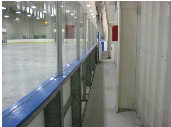
D13 perimeter corridor with access to player boxes
