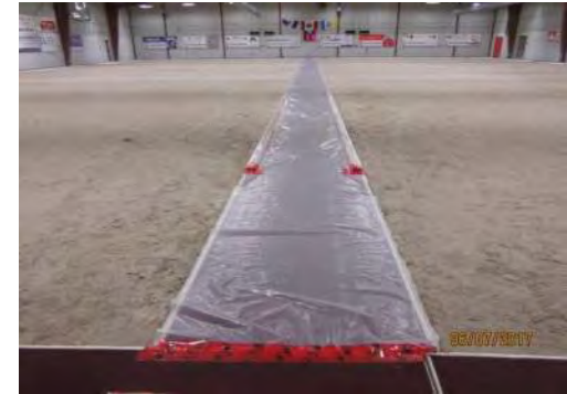
D15 Curling Rink (accessed from Lower Level): Central aisle does not have space to turn around for users of mobility aids.
