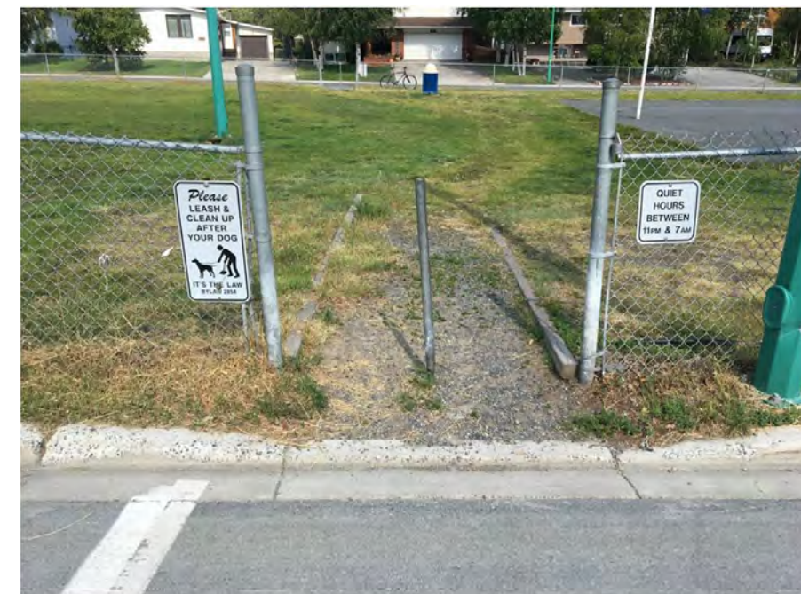
entrance gateway with post intended to block vehicles
