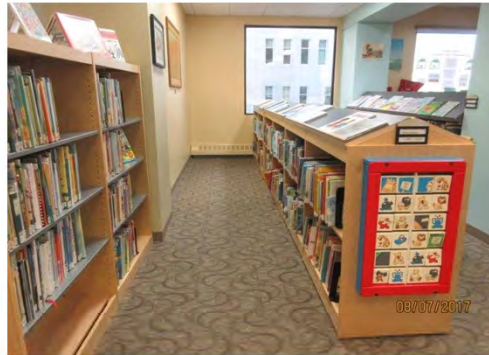
D32 Kids Section: Circulation for users of mobility aids is limited, with no turning space provided at one end.
