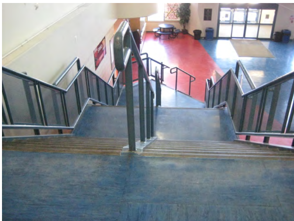
B18 Main stairway from top
