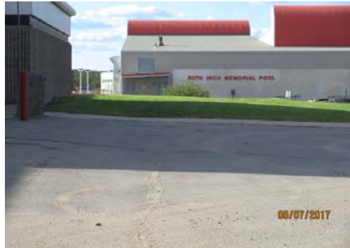
A7 Approach to main entrance (west side).
