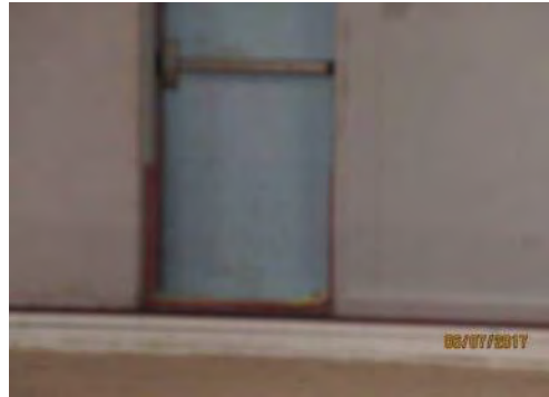
C8 Exit from Curling Rink (typical): Stepped transition only.
