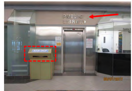
B12 Book Return, elevator lobby (ground floor, mall): Identification sign has large print and suitable colour contrast. Overhead library identification signage does not have strong colour contrast.
