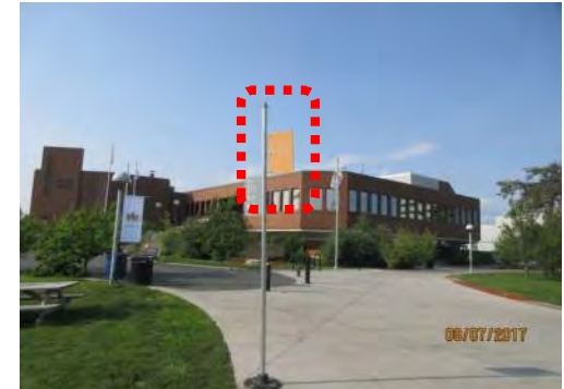
A3 Approach to City Hall from south west side, off of 49th Street. Post-mounted directional signage is provided.
