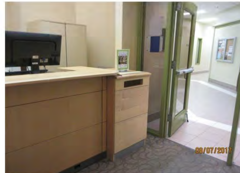
B23 Main entrance, circulation desk: No lowered counter is provided. Book deposit slot is accessible, however, identification signage would be beneficial for all users.
