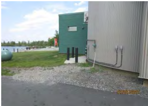
D63 Somba K'e Service Building (exterior): Approach from driveway at rear of building.
