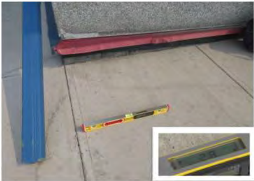
A19 Main entrance area: Running slope of sidewalk is suitable at 2.8%.
