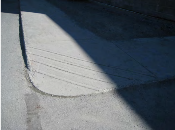
A7 Curb ramp (typical)
