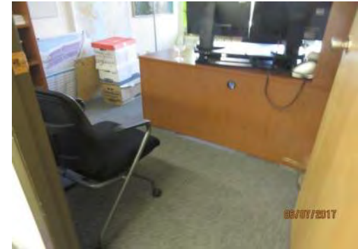
D51 2nd floor (south east side): Generally, work areas would require reconfiguration of furniture & equipment to address accessibility.
