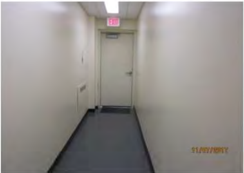
B32 1st floor, View of corridor to exit door(south west side): Level access is provided on exterior side.
