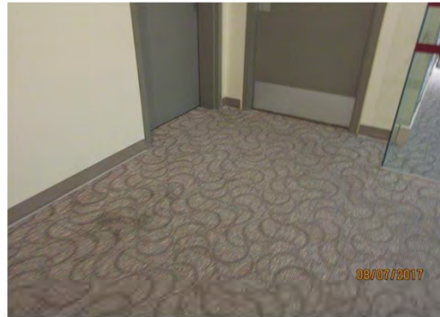
B68 Women's Accessible Washroom: View of approach to entrance, off of enclosed area.
