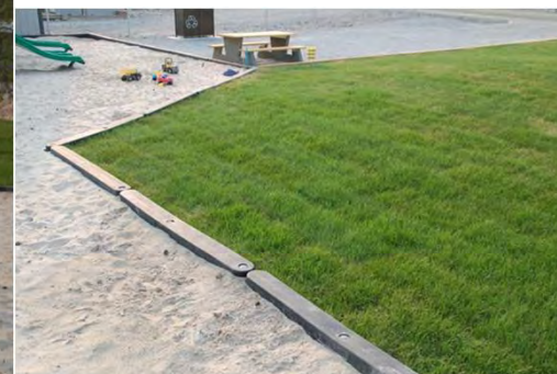
level change with no ramp threshold over rubber retaining edges
