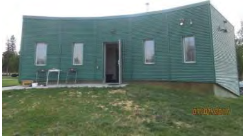
D60 Somba K'e Service Building (exterior): No building identification signage was identified at time of audit.
