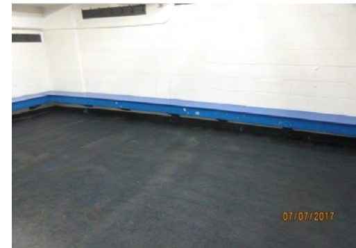
D36 Change Room #4 (Lower Level, north side).
