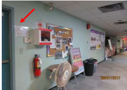
C1 Fire safety plans are provided adjacent to exits. Information boards are typically mounted too high and posted information is cluttered. AED cabinet is mounted too high, with no cane detectable leading edge.
