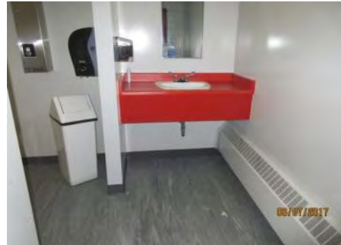
B44 Main Floor (adj. to secondary entrance): Women's Washroom. Identified as accessible through door signage but it is not accessible.
