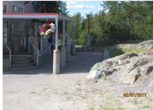
A2 Approach to facility: No separate public sidewalk is provided, as users must walk along drive aisle. Exterior site and facility identification signage is limited. Main entrance is not clearly marked with signage, however, design is prominent.
