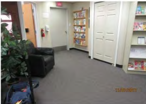
B13 2nd floor, entrance lobby & reception area: Circulation is suitable. No elevator access is provided to 2nd floor.
