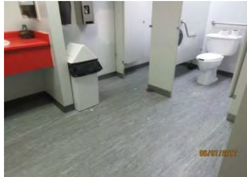
B38 Women's Washroom (adj. to entrance): Identified as accessible through door signage but it is not accessible. No accessible lavatory.
