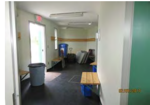
D90 Somba K'e Service Building (interior): Many interior areas are used for storage. Clear floor space is limited.
