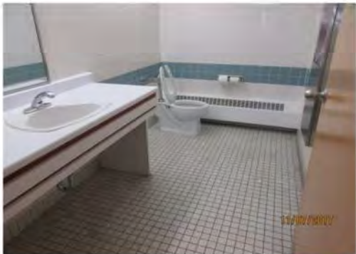
B36 2nd floor, interior view of Washroom #2: No accessibility features identified. However, 2nd floor is not accessible.
