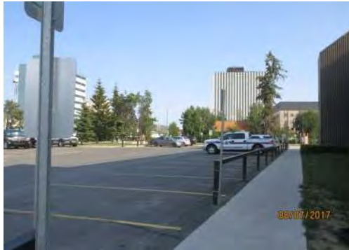
A13 View of staff parking lot (east side of site): No accessible parking spaces are provided.
