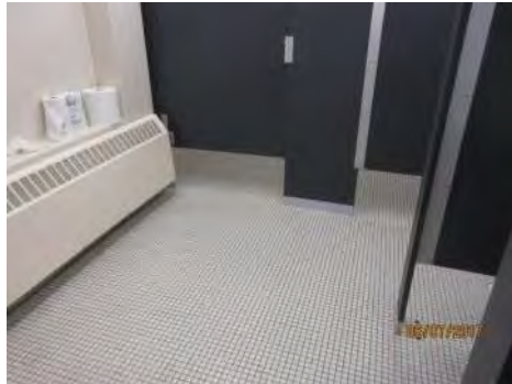
B91 Men's Accessible Washroom, main floor: Interior features are non-compliant. Limited interior floor space.
