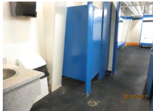
D35 Shared Washroom, Change Rooms #3 & #4 (Lower Level, north side): Limited interior floor space for shared facilities.
