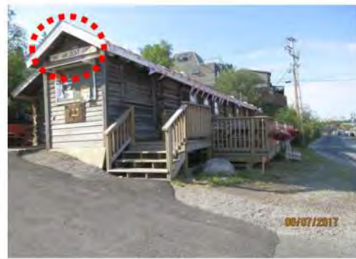
A11 Adjacent roadway and approach to main entrance and deck has significant slope. Overhead building identification signage is mounted on façade but is generally not highly visible.
