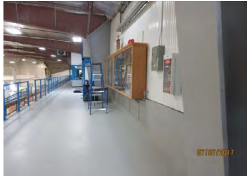
D7 Corridor & Viewing Area (Upper Level, south side): Display cabinet projection.
