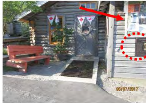
A8 Main entrance is not accessible due to elevation change and high threshold. A heritage display plaque is provided adjacent to main entrance.
