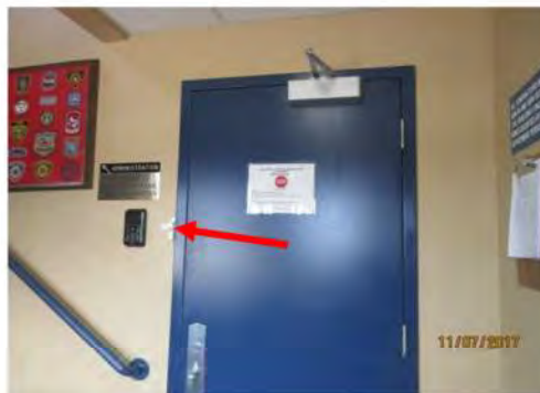
B8 Main entrance vestibule: View of door to 1st floor Offices (Operations), Kitchen and Dormitory. Door bell, operating controls and signage are mounted too high.
