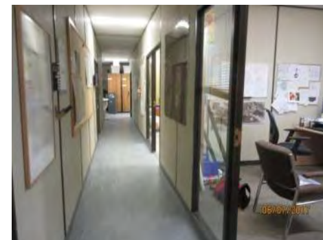
B72 Corridor, main floor (south side): Suitable clearance is provided and corridor is well maintained.
