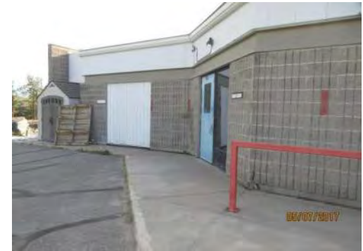
A9 Approach to secondary entrance: Clear width of sidewalk is reduced significantly by guardrail.
