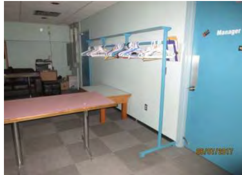
B8 Approach to Manager's Office, upper level. Office was locked at time of audit.
