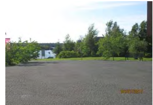
A24 Approach to waterfront, west side of site. Stamped concrete / brick paver surface is generally in very good condition.
