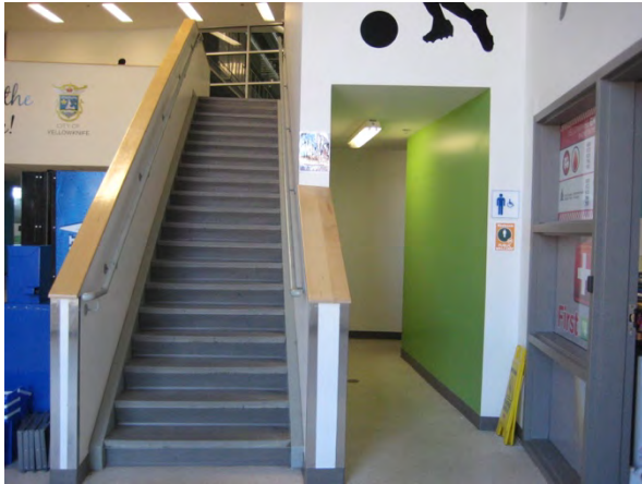
B14 doorless access to washroom main level to right of stairs (typical)
