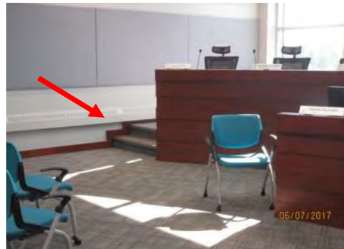
D14 Council Chamber: Approach from public gallery. Step access only.
