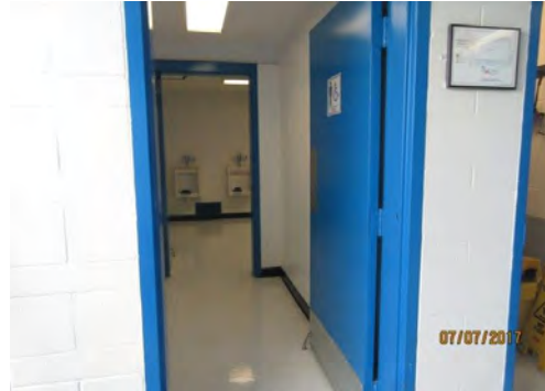
B26 Men's Accessible Washroom (Upper Level): Entrance doors have limited clear width but typically suitable for an existing condition. Door mounted signage is not accessible. No power door operators are provided.
