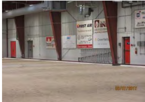
D19 Curling Rink: View of rink surface which was under maintenance.
