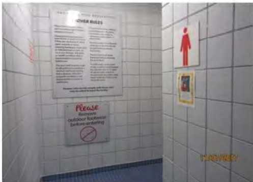
D10 Entrance corridor to Men's Change Room . Circulation clear width is typically limited for larger wheeled mobility aids. Identification signage is not accessible.
