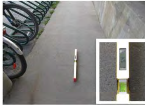
A14 Approach to main entrance from accessible parking spaces (intermediate section): Running slope is on-compliant at 5.4%.
