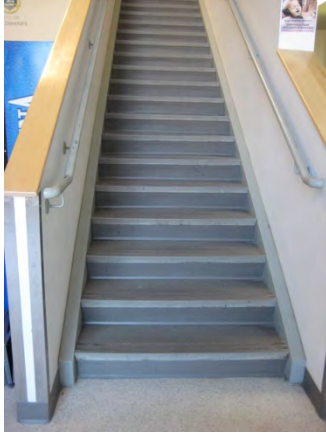
B10 stairs from main lobby to upper lobby area
