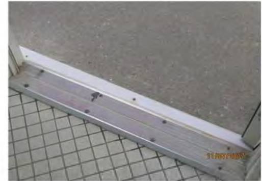
B3 Main entrance: Level access is provided. Beveled threshold is suitable.
