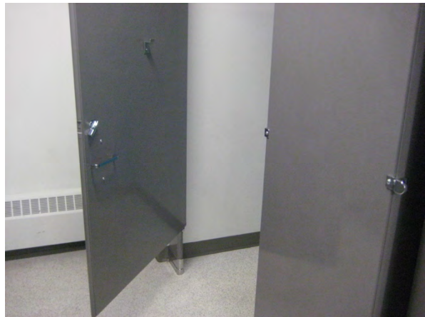
B17 accessible toilet stall door main level female washroom
