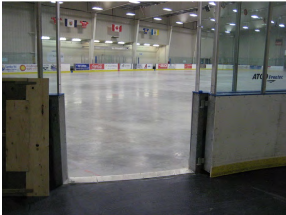
D12 access to ice surface
