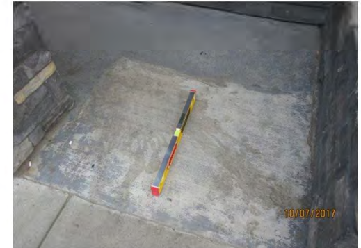
A6 Ramp: Typical running slope of bottom landing is suitable at 3.1%.
