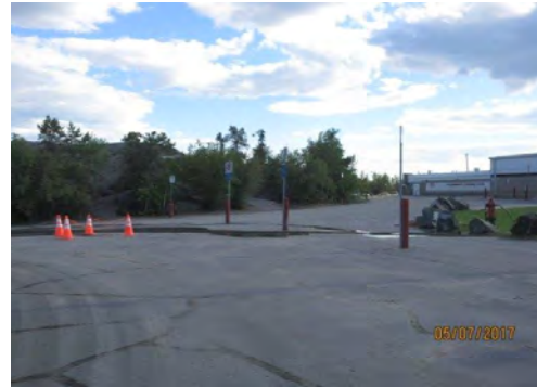
A2 Approach to main entrance, from west side. Parking spaces are not clearly marked (e.g., pavement line markings), including accessible parking.
