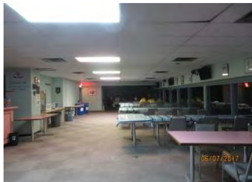
B10 View of viewing / assembly / dining area, upper level.
