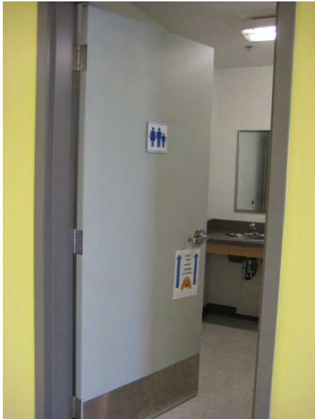
B20 washroom in play area
