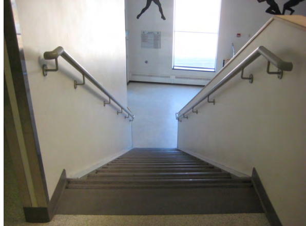
B11 stairs from upper lobby to main lobby
