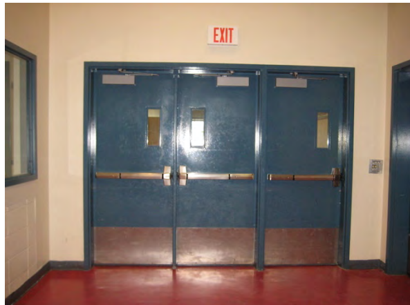
C4 Exit doors leading into upper lobby from arena viewing area.
