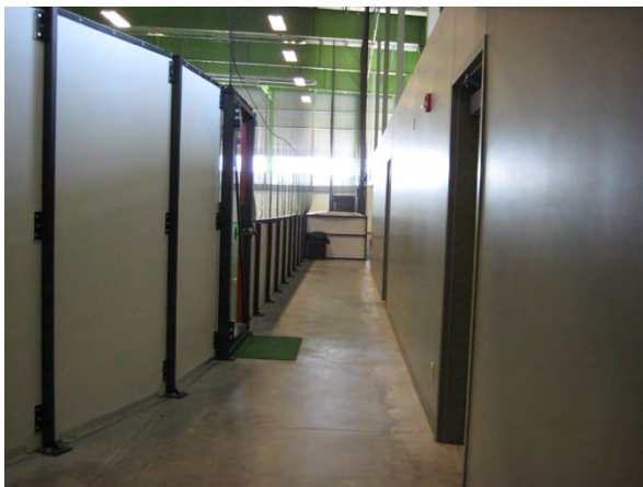
D11 corridor at perimeter of soccer fields
