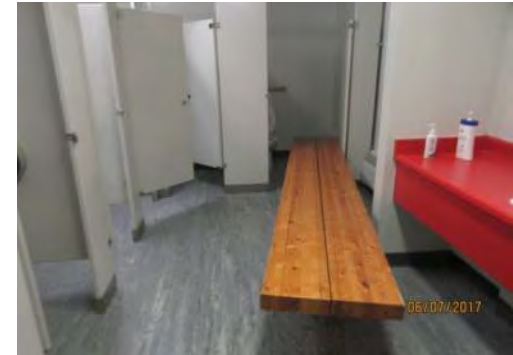
D39 Women's Changeroom (Lower Level): Washroom stall layout / configuration.
